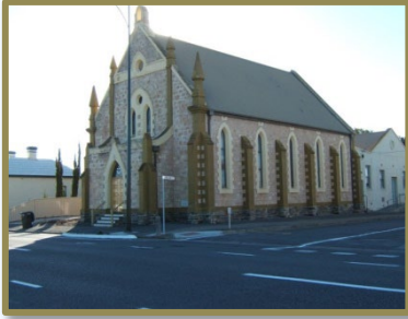
Manthorpe Memorial church. One of several designed by Charles Eaton Taplin
